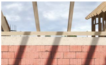
Wooden beams adjustment
